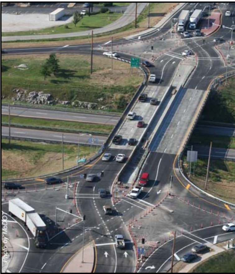
Traffic crisscrosses at either end of the bridge, so instead of making hard left turns, drivers veer to the left for access.
