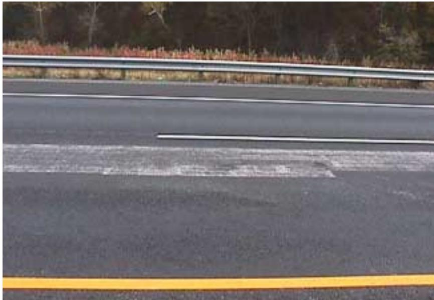
**Picture 9 – Grinding to Correct Flushing in Wheelpath**
