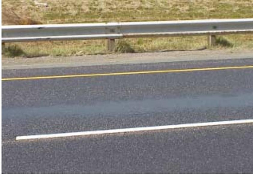
**Picture 8 – Flushing Isolated In Wheelpath After Placement**
