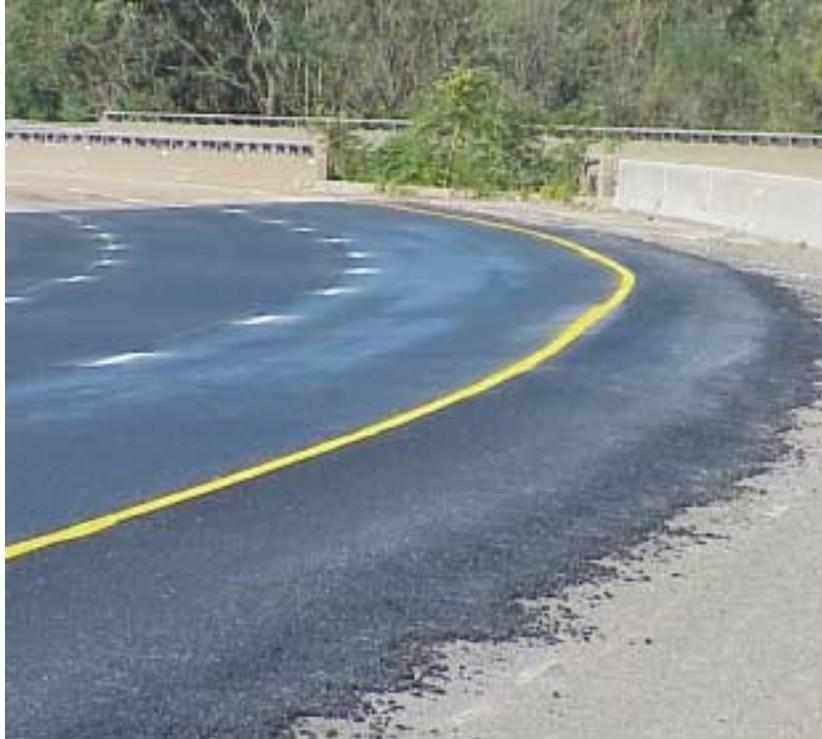
**Picture 6 – Flushing Pavement – Failure to “Waste” First Loads**
