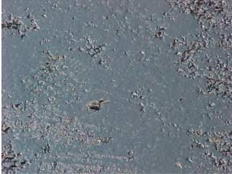
**Picture 7 – Close-Up of Flushing – Excessive Moisture in Mineral Filler**
