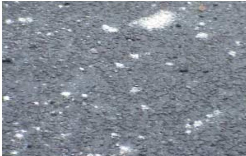
**Picture 12 – Fractured Aggregate – Surface**
