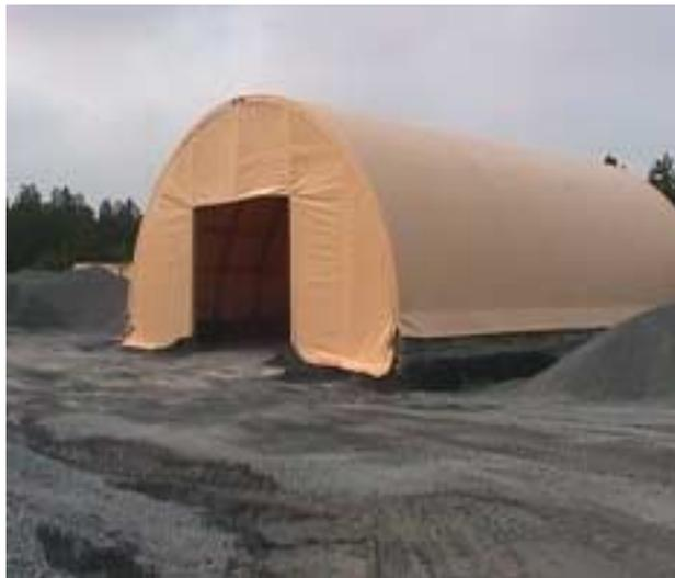
**Picture 3 – Storage Facility to Protect Mineral Filler**
