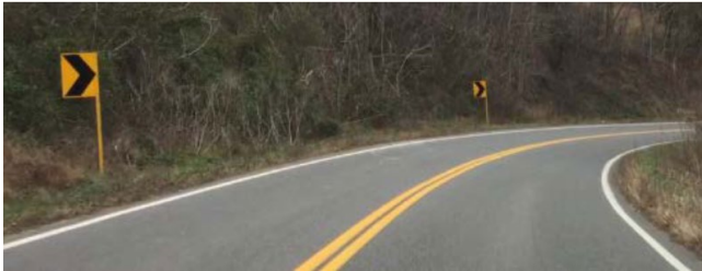
Retroreflective material on chevron posts.
